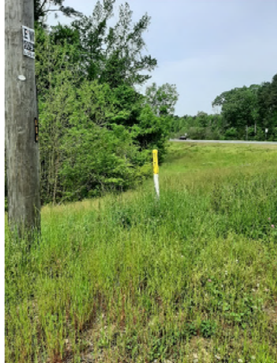
Gas line (SW quadrant of intersection)
