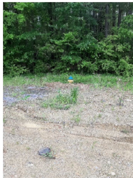
Water lines/Hydrant (SE quadrant of intersection)
